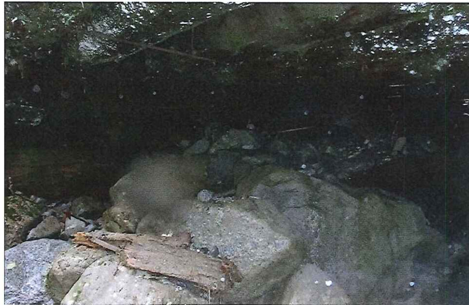
CK2267 Right Abutment
