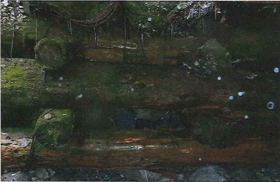
CK2267 Left Abutment
